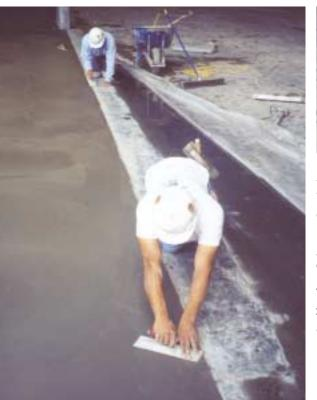
to ensure that the plate does not restrain lateral movement while still transferring the total vertical load. The original design called for traditional square dowels and clips, but DPI was convinced to use the diamond plate dowels upon learning that Fricks had become advocates of the new system because of its many advantages.
